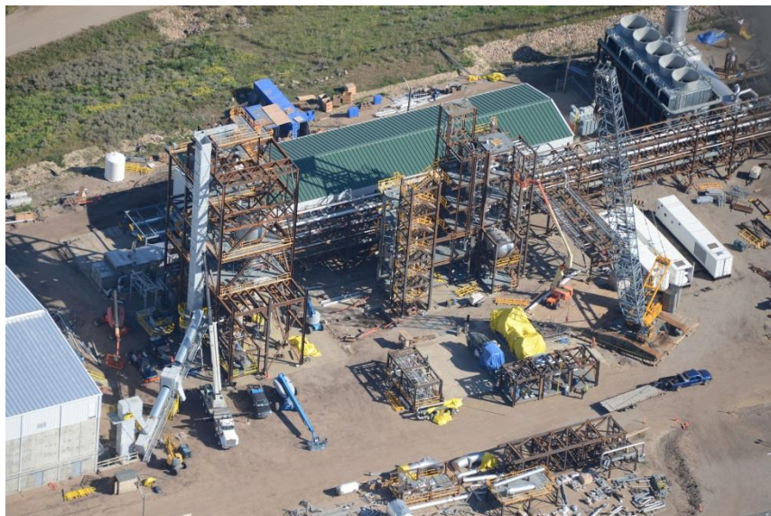
Figure 2. VVANERO (Enerkem/GreenField partnership) plant in Varennes under construction
