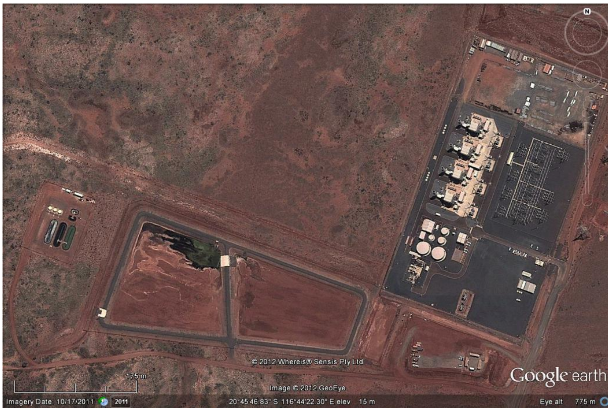
Figure 4. Muradel site - three raceway ponds to the west of Yurralyi Maya power station
