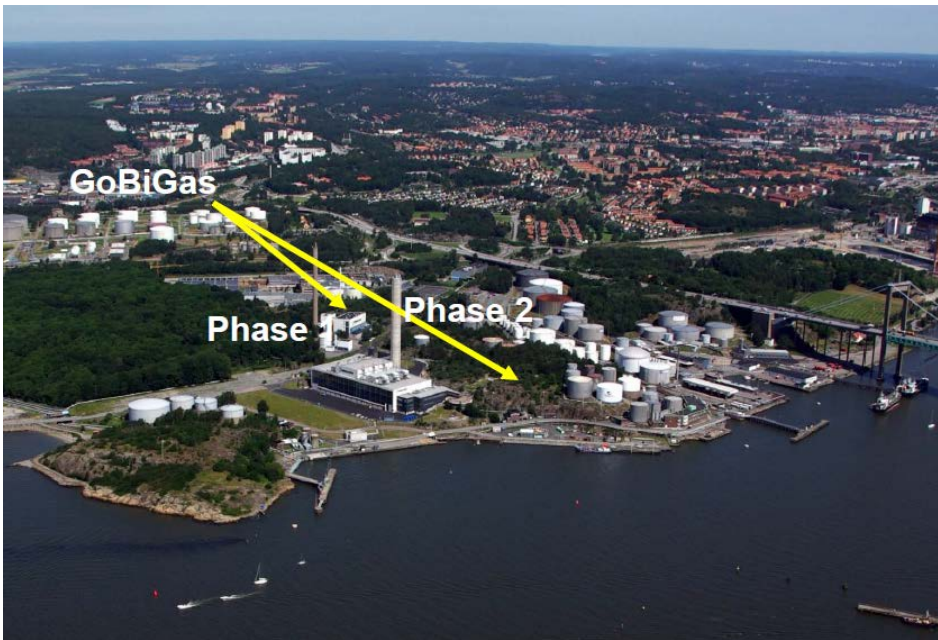
Figure 8. Photo of the Rya location showing the Gobigas plants. Reference: Göteborg Energi.
