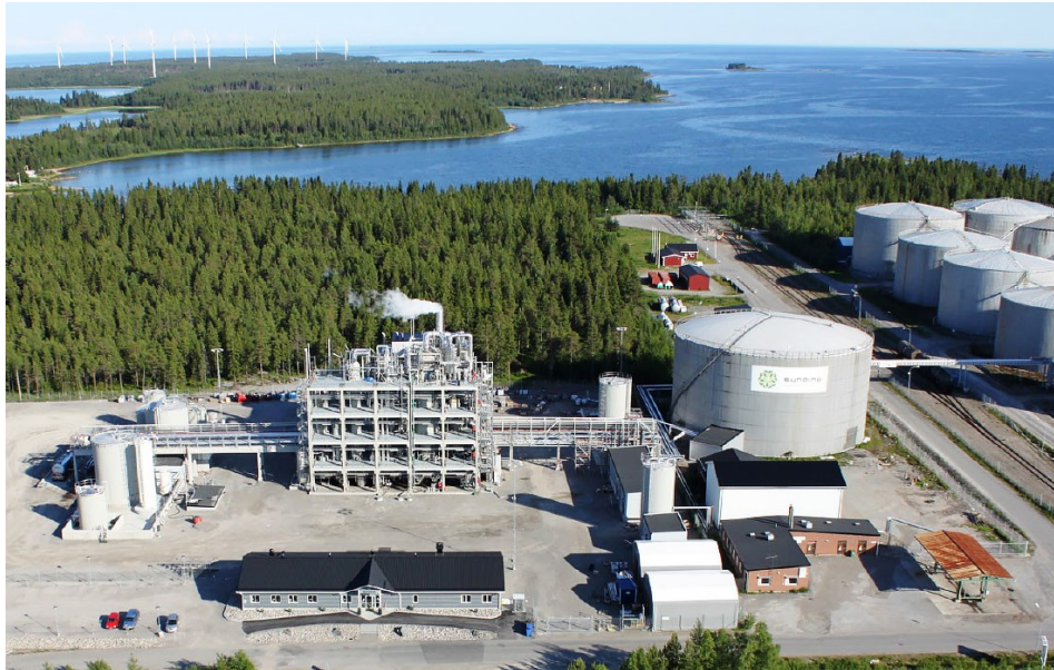
Figure 3. SunPine production plant in Piteå. Reference: SunPine.
